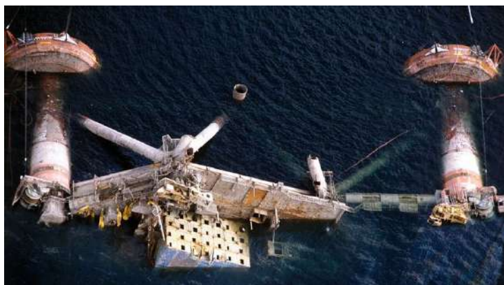
Figure 12-4: The Alexander L. Kielland platform capsizing
