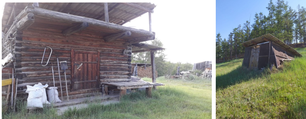
Figure 1. The two types of buluus : with storage house and shed. It is done to protect the permafrost. A good example of Sakha cooperating with and conserving the permafrost. Credit: Maria Burnasheva, Vasilii Burnashev.
