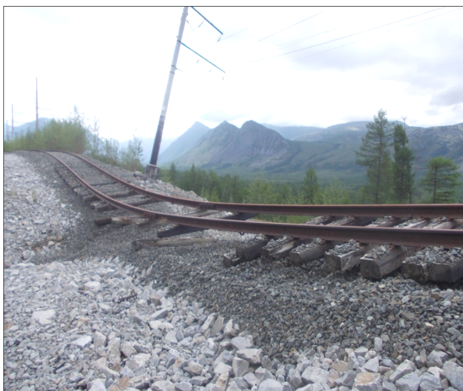
Figure 5. Disturbances in the zone of Chara-China Road due to the development of dangerous geocryological processes (photo by I. Chesnokova, 2016).
