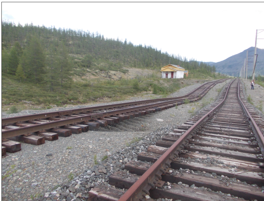
Figure 3. Disturbances in the zone of Chara-China Road due to the development of dangerous geocryological processes (photo by D. Sergeev, 2016).
