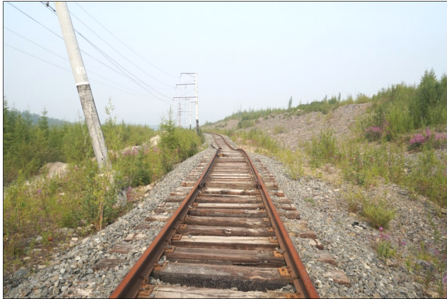
Figure 2. Disturbances in the zone of Chara-China Road due to the development of dangerous geocryological processes (photo by I. Chesnokova, 2016).
