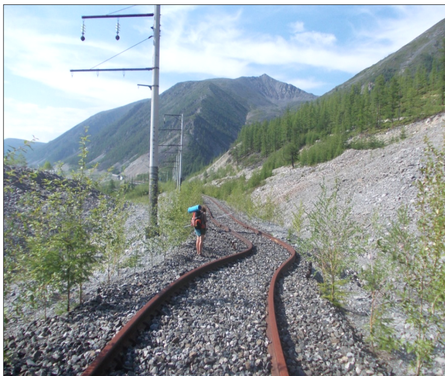
Figure 4. Disturbances in the zone of Chara-China Road due to the development of dangerous geocryological processes (photo by I. Chesnokova, 2016).
